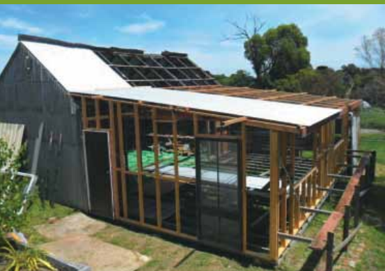
Renovation of old barn
